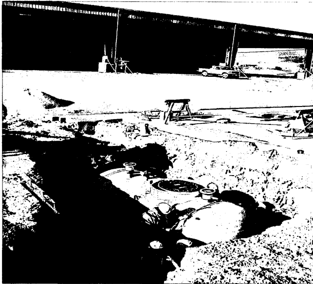
Oil Water Separator Unit
