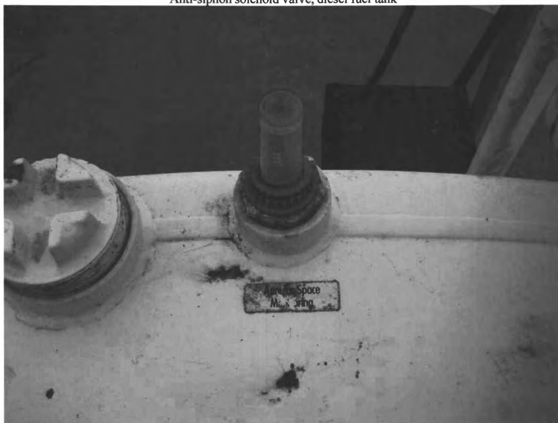
Tank Interstitial Monitor
