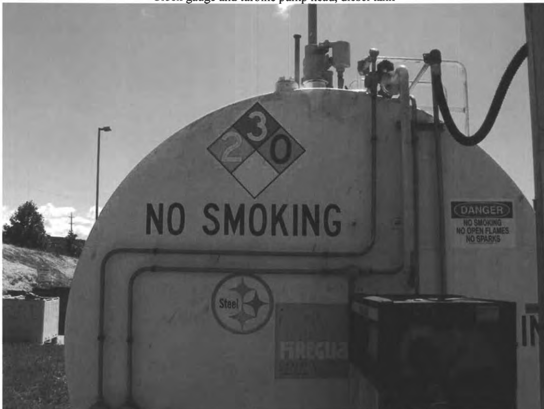
End view of gasoline tank showing NFPA placard
