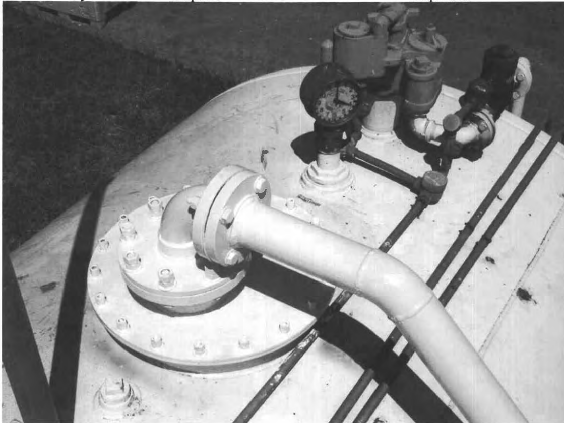
Clock gauge and turbine pump head, diesel tank
