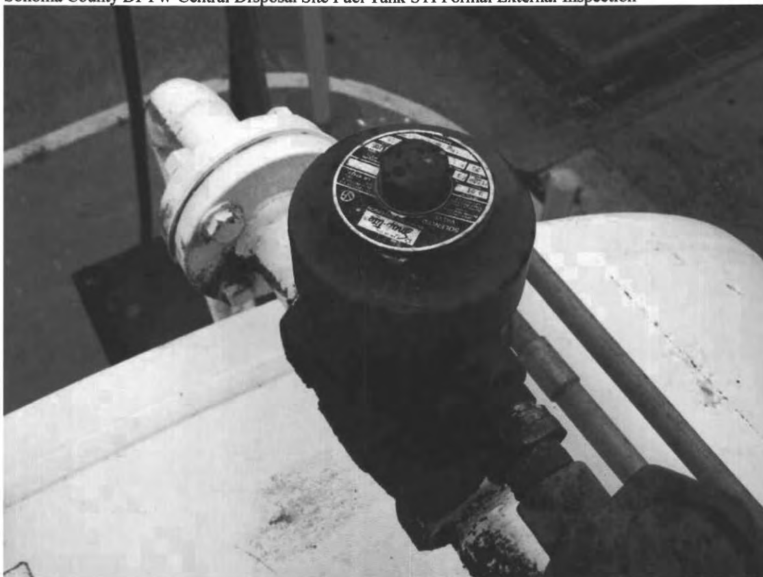
Anti-siphon solenoid valve, diesel fuel tank
