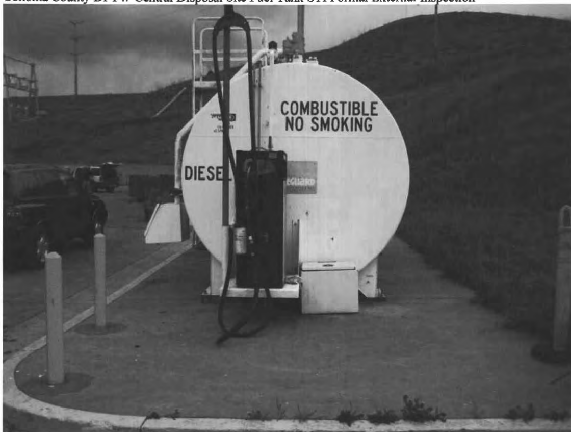
End view of tank, diesel side. Concrete pad slopes to left, then is directed to OW Separator
