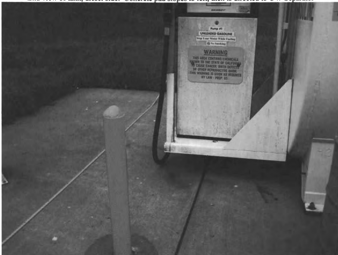
Gasoline dispenser; elevated dispenser platform allows for immediate detection of piping leaks
