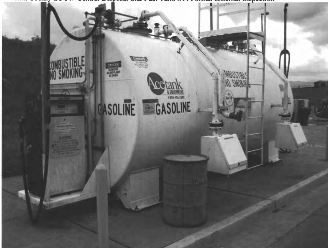
Fuel Tank, gasoline end with integrated dispenser
